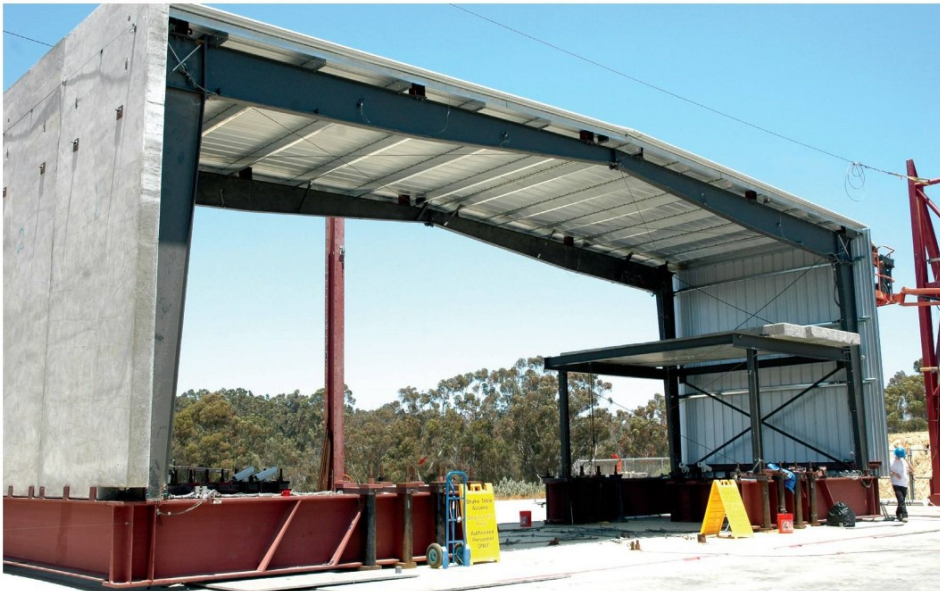
Metal building with heavily loaded mezzanine and concrete sidewall.
