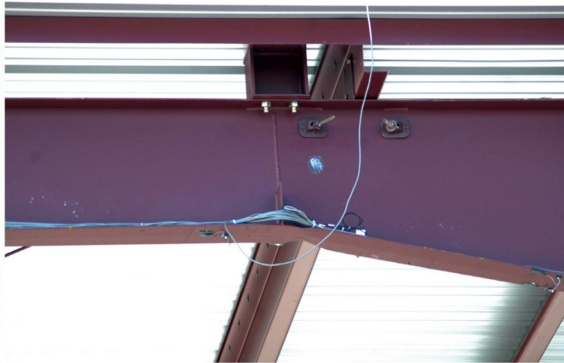
Metal building with heavy concrete walls.
