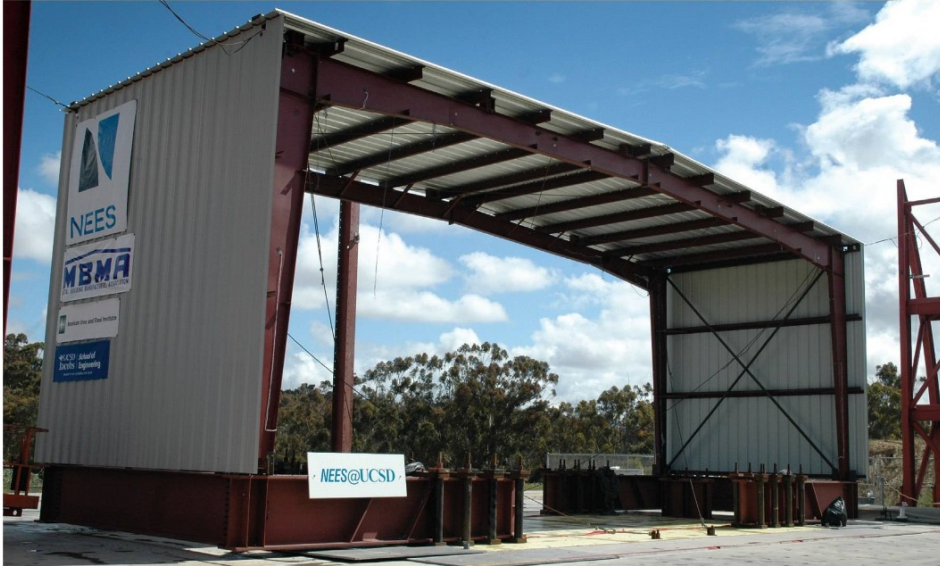
Metal building with metal sidewalls.
