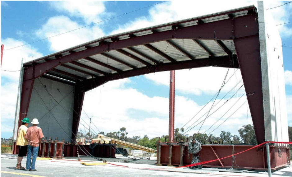
Metal building with heavy concrete walls.
