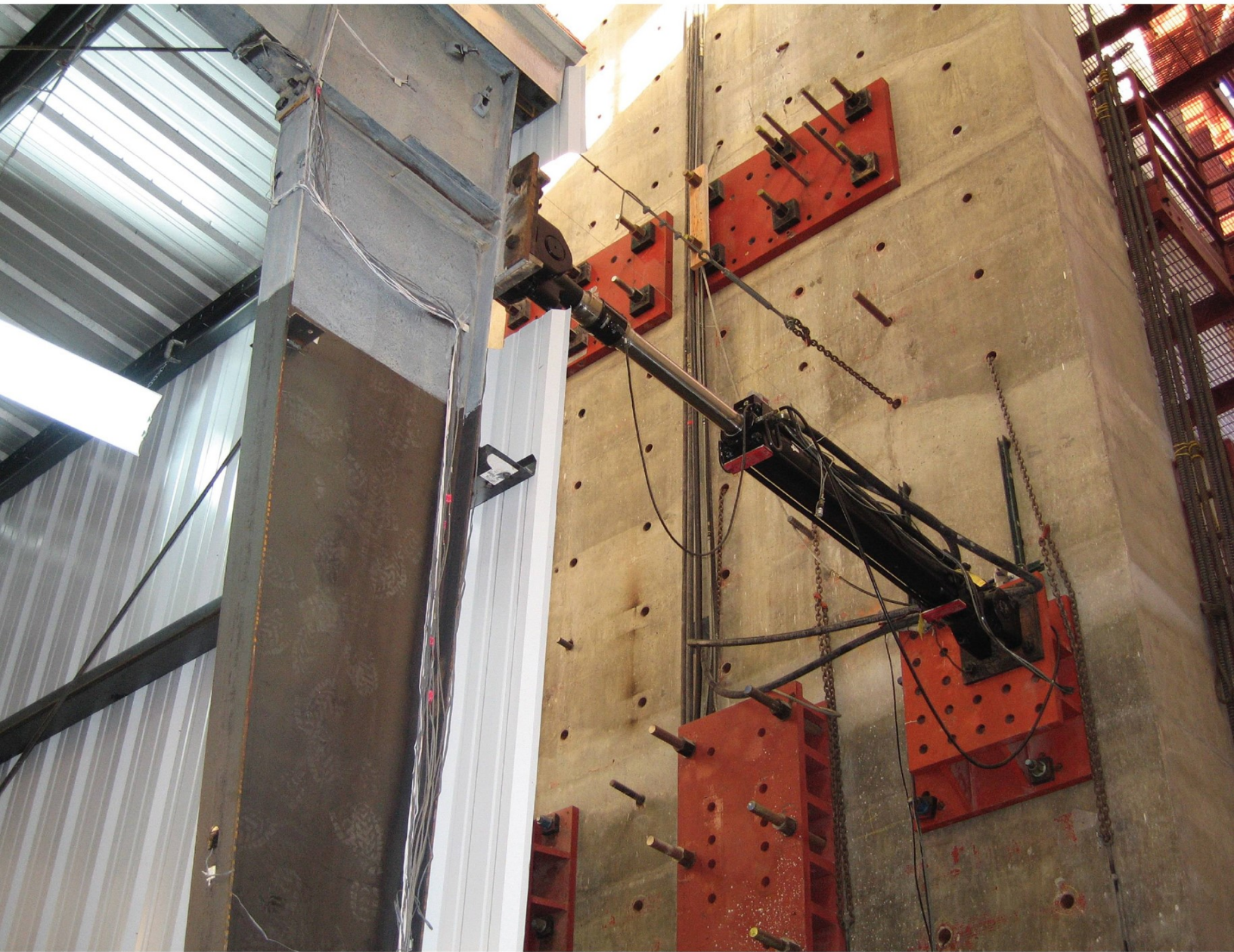
Photo 1: Cyclic Test. One of the load actuators used to alternately push and pull the metal building system frame back and forth to assess its behavior and ductility.
