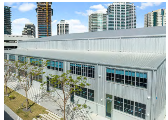
Grove Bay Marina Hangars • Coconut Grove, FL
