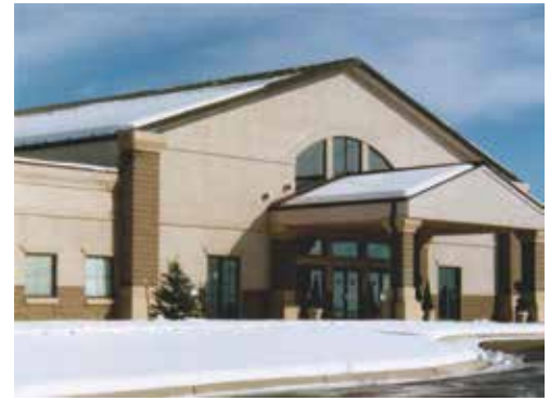
Metal building gable roof snow loading. Courtesy of the Metal Building Manufacturers Association.
