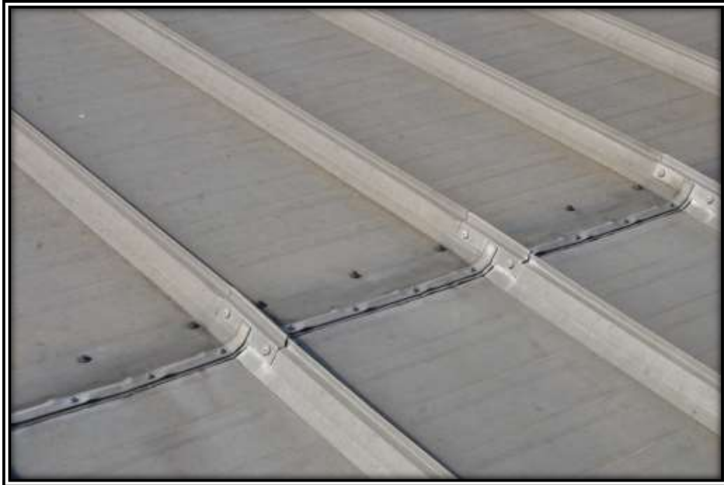
Photo B: This thirty year plus trapezoidal standing seam roof still performing.
