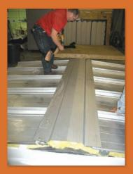
A volunteer installer puts the finishing touches on this ridge installation just prior to performing an air leakage test. to save energy for metal building owners.
