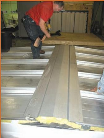
A volunteer installer puts the finishing touches on this ridge installation just prior to performing an air leakage test.
