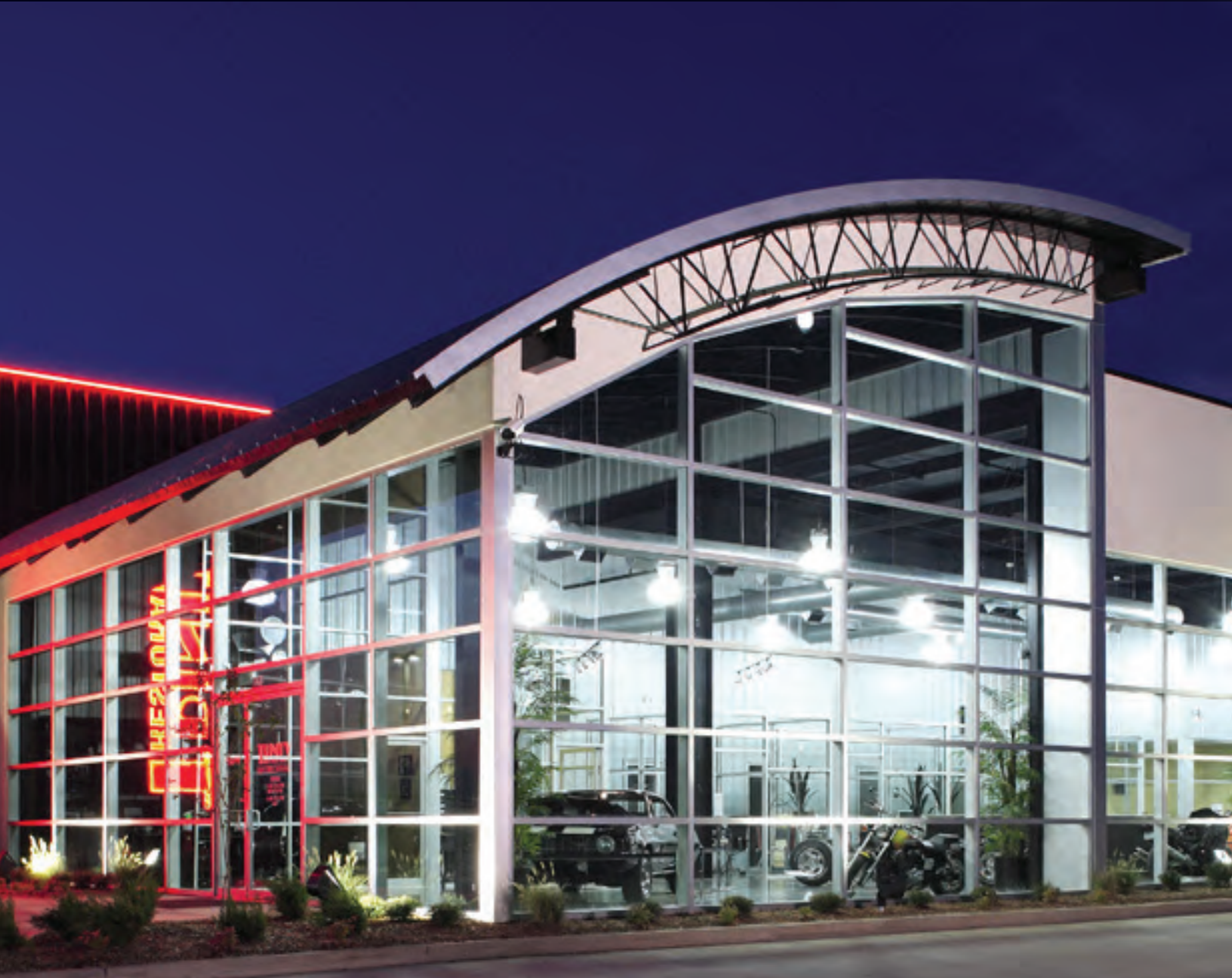
Trinity Restoration • Tulsa, OK
