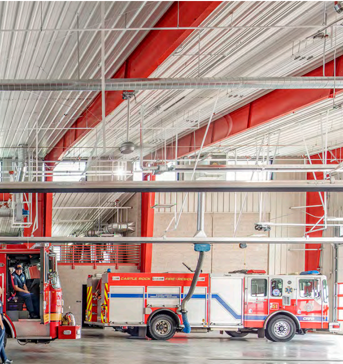
Castle Rock Fire Station #152 • Castle Rock, CO
