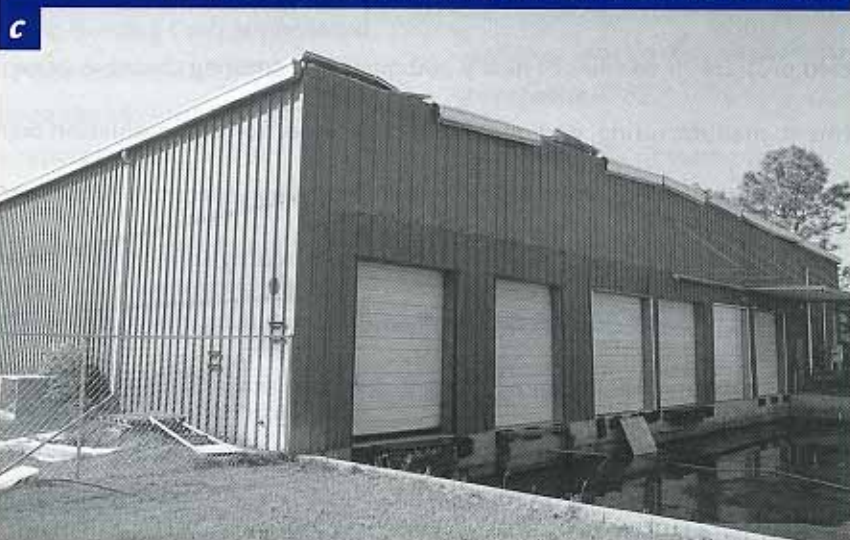
Note that the building designed to more recent code in Opal only suffered damage to canopy and edge flashing.
