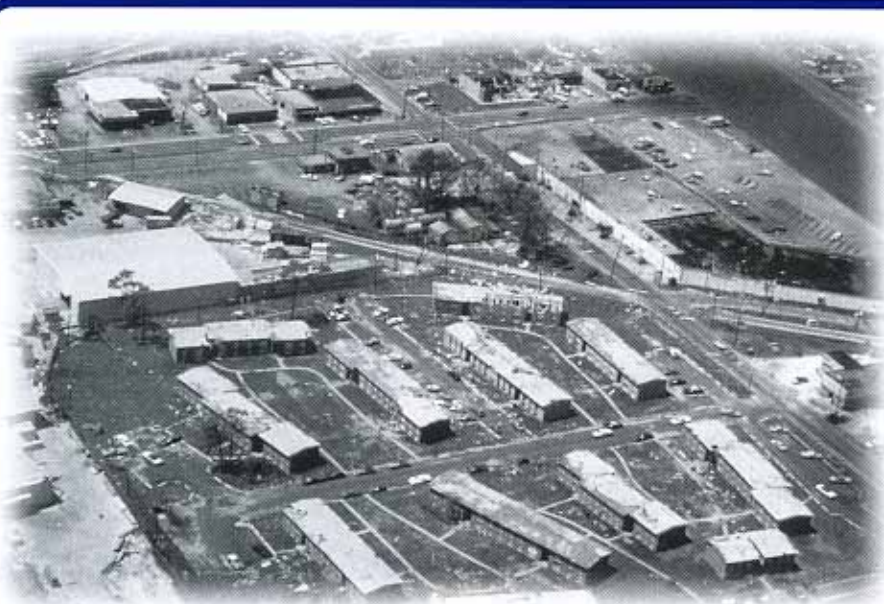
Photo 3: Hurricane Elena Observation – Large cross-section of metal buildings and metal roofs designed to various codes due to their apparent age. Newer buildings show little or no damage.
